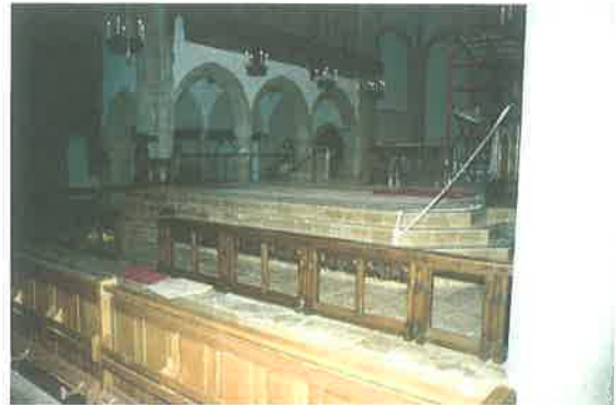
New chancel floor and communion rail (103)
