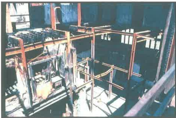
Basement viewed from the first floor (45)
