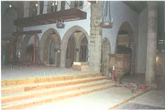
Chancel floor is raised 2 feet (93)
