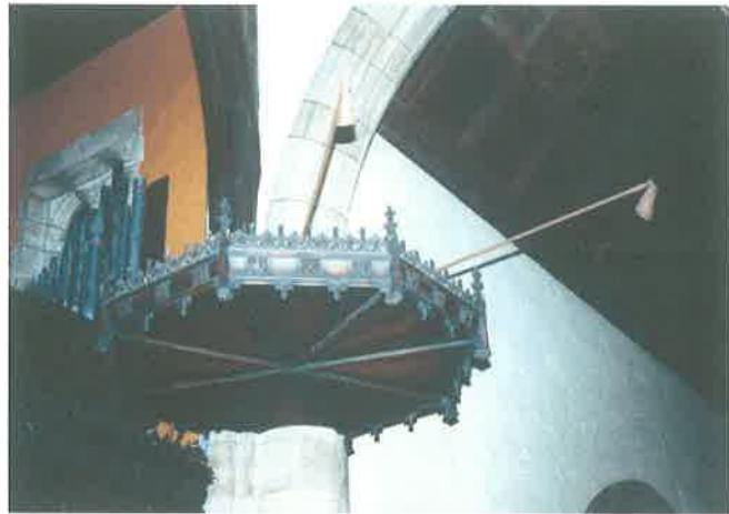
Pulpit canopy prior to renovation (28)
