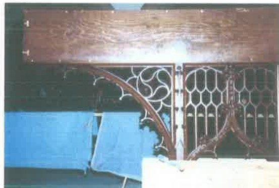
Sections will wrap new Rood Beam (100)
