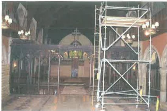
Rood Screen being readied for removal (64)
