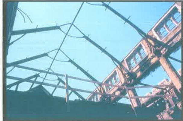
Roof, viewed from second floor (46)
