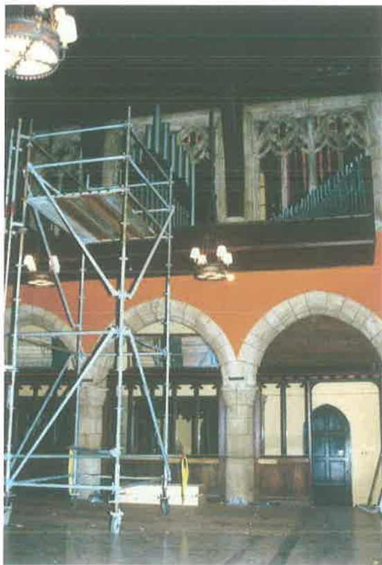
Organ pipes being removed (66)
