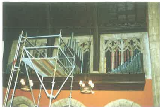
Organ pipes being removed (65)
