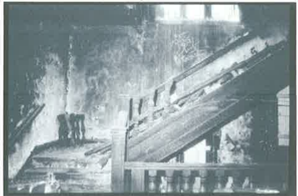
Main staircase in Parish House (44)
