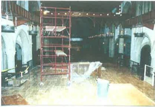
New floor installed in chancel (except elevator) (102)
