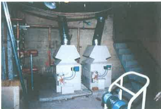
A new heating plant was installed (95)
