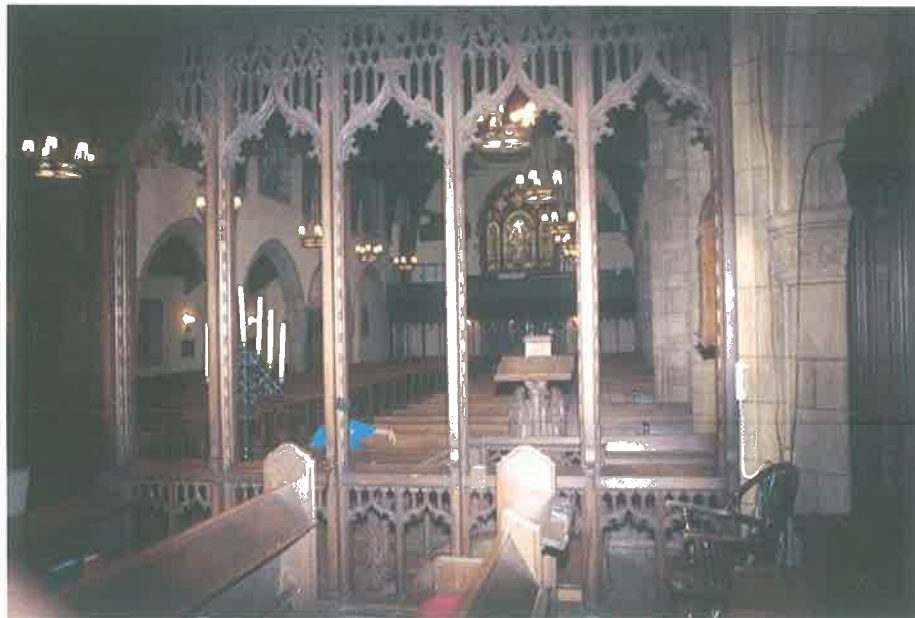
Facing west from the north side of the choir loft, through the Rood Screen and past the Lectern. The Rood Screen was removed and replaced by a Rood Beam, built from the remains of the Rood Screen and placed around a new steel girder installed for seismic reasons during the renovation in 1991. (29)
