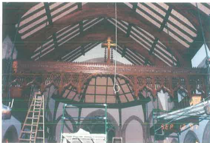
Sections were pieced together to cover new seismic beam to become the new Rood Beam (101)
