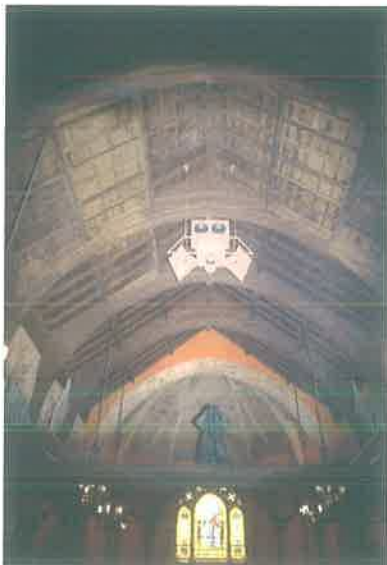
Ceiling prior to renovation (25)
