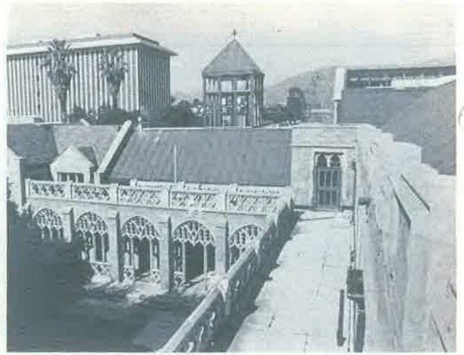
LOOKING NORTH TO THE TOWER
