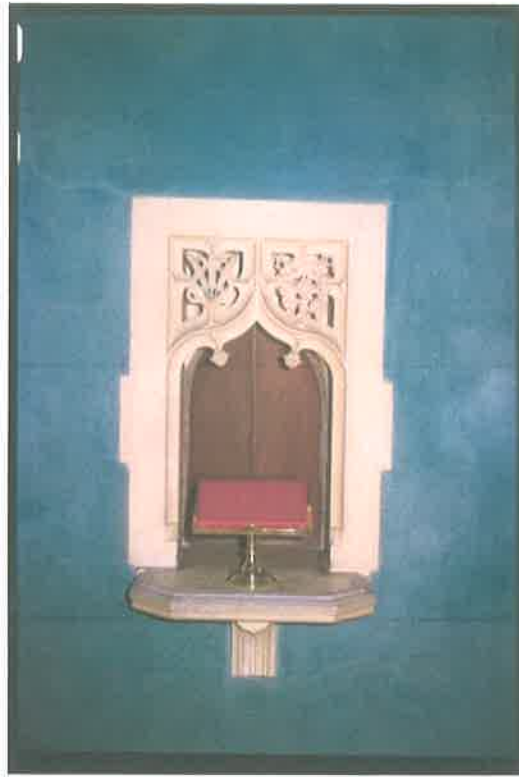
The Credence Shelf (next to the High Altar) – Erected by Miss Catherine Ahern in memory of Miss Elizabeth Remsen. The shelf consisted of a plaster niche and shelf for the Sacraments. The carved decoration was a Gothic tracery arch, wheat and flowers. The doors on the back of the shelf opened into the Ambulatory, across from the Sacristy. (190)
