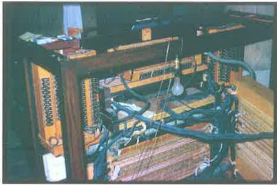
Console being rewired (37)
